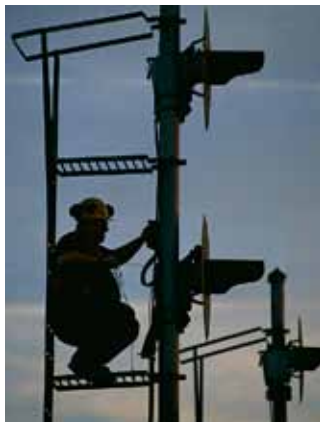
A Union Pacific signal maintainer examines the moving parts behind a signal that gives instructions to engineers. Howard Ande
