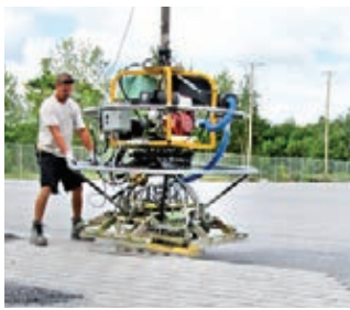
Techo-Bloc offers the TB-100si, a machine specially designed for the installation of Inflo permeable pavers.
